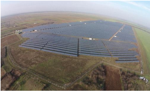
Fig. 3 Photovoltaic power plant
