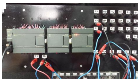
Fig. 15. Connect wires for the second application
